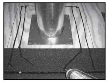
Figure 10.20 Apply Sealant
